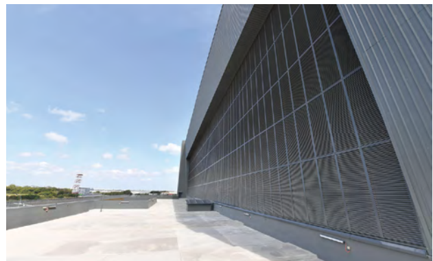
Large-span louvres located at the back contribute to natural ventilation of the building.
