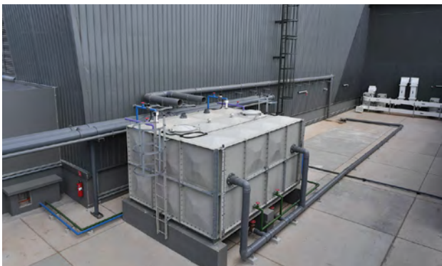
Rainwater is harvested and recycled for general washing, auto-irrigation of the hangar's green roof, and flushing of toilets, so as to conserve potable water.
