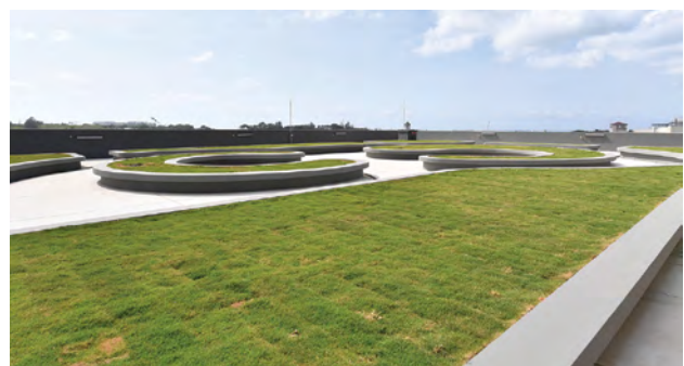
The green roof acts as an insulation layer to reduce solar heat gain into the building.
