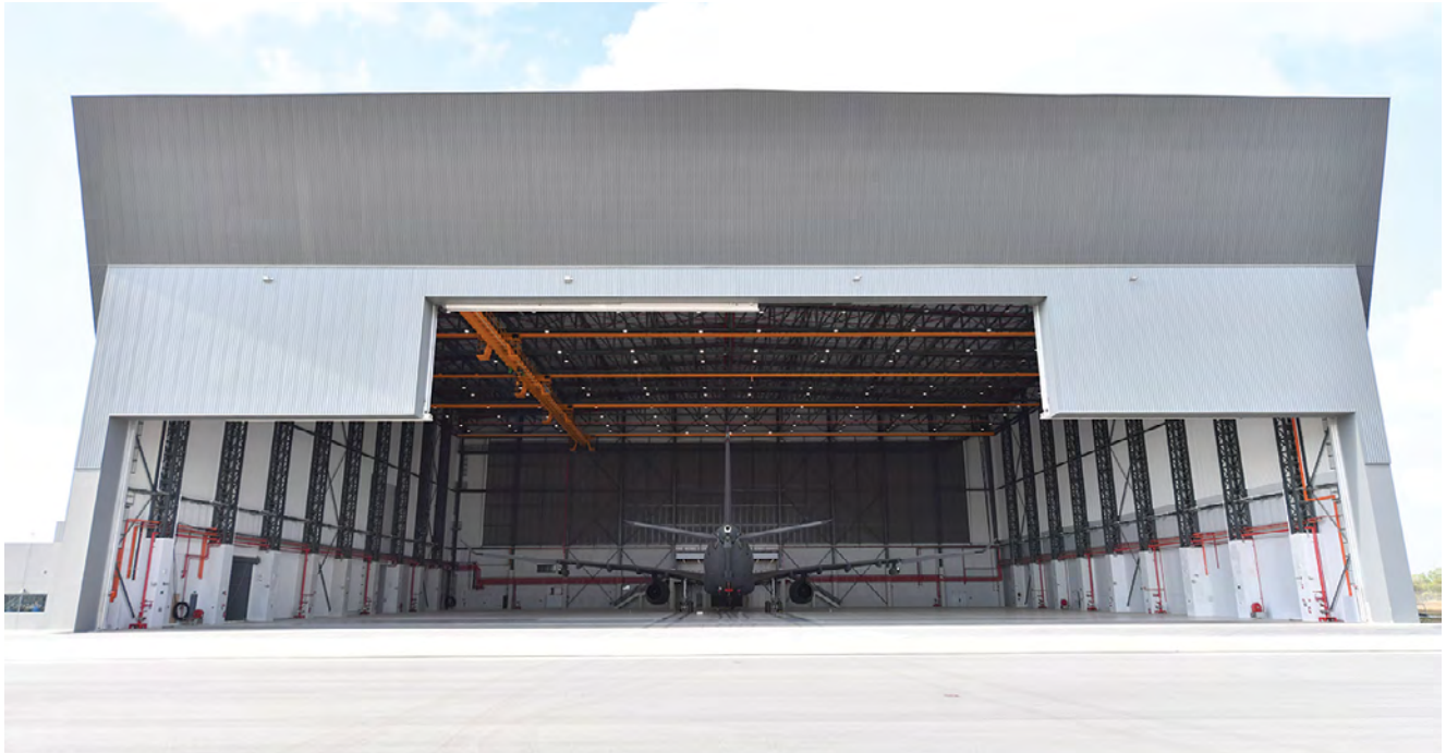
The hangar for the Republic of Singapore Air Force's (RSAF) A330 Multi-Role Tanker Transport (MRTT) aircraft is located at Changi Air Base (East).
