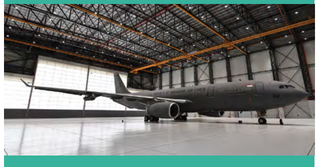
The hangar with the panelled fabric doors lifted (image above) and lowered (image below). The translucent fabric doors allows natural light transmission into the building, thereby reducing the artificial lighting requirements.
