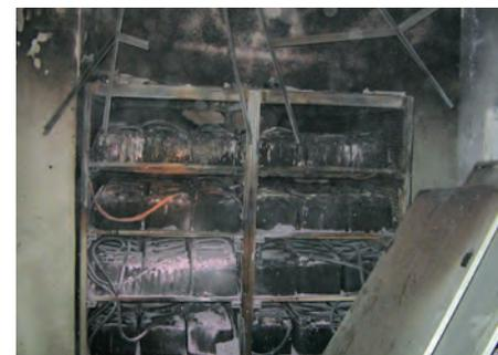
Figure 1. Burnt UPS batteries
