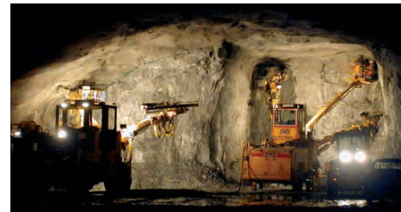
Figure 4. State-of-the-art drilling jumbos in operation
